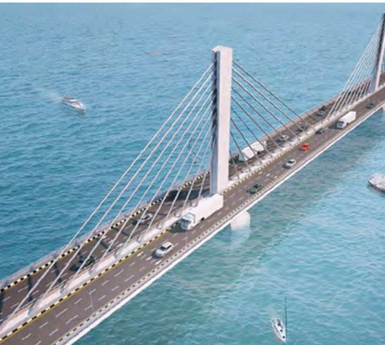
A semi-fan system of single-plane cable stays connects the superstructure to two 55-m-high pylons.
