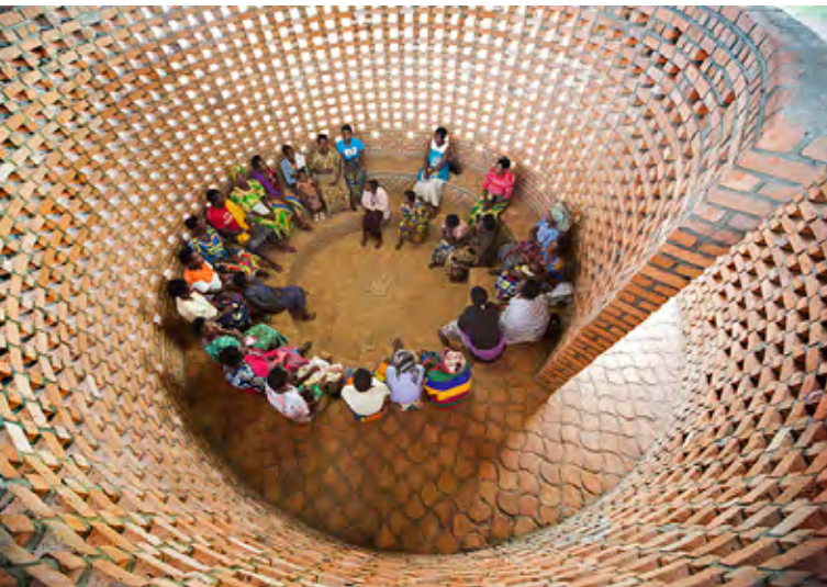
Perforated classroom walls enable passive cooling and solar shading.
