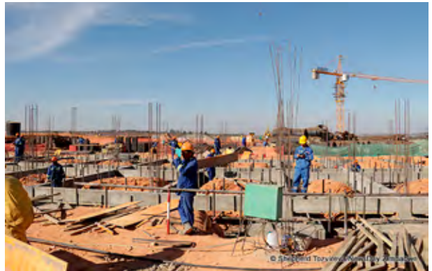
Work on the new PPC Zimbabwe plant at Msasa has started.
