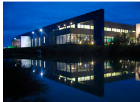
Page 24 - Industrial architecture and a passion for concrete characterise architect Thierry Bogaert's work. He is a headline speaker at TCE East Africa.
