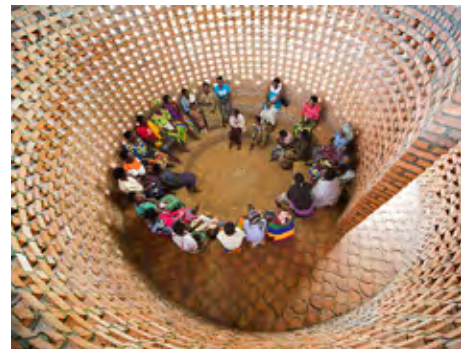
Page 8 - At the Women's Opportunity Center in Rwanda, perforated classroom walls provide passive cooling and solar shading.
