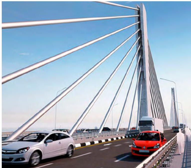
The deck is a prestressed box girder 32 m wide accommodating a six-lane dual carriageway and two sidewalks.
