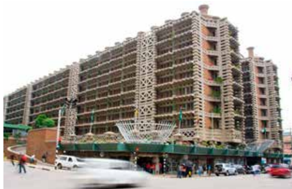
The Eastgate Centre's passive cooling system was inspired by the way termite mounds stay cool.
