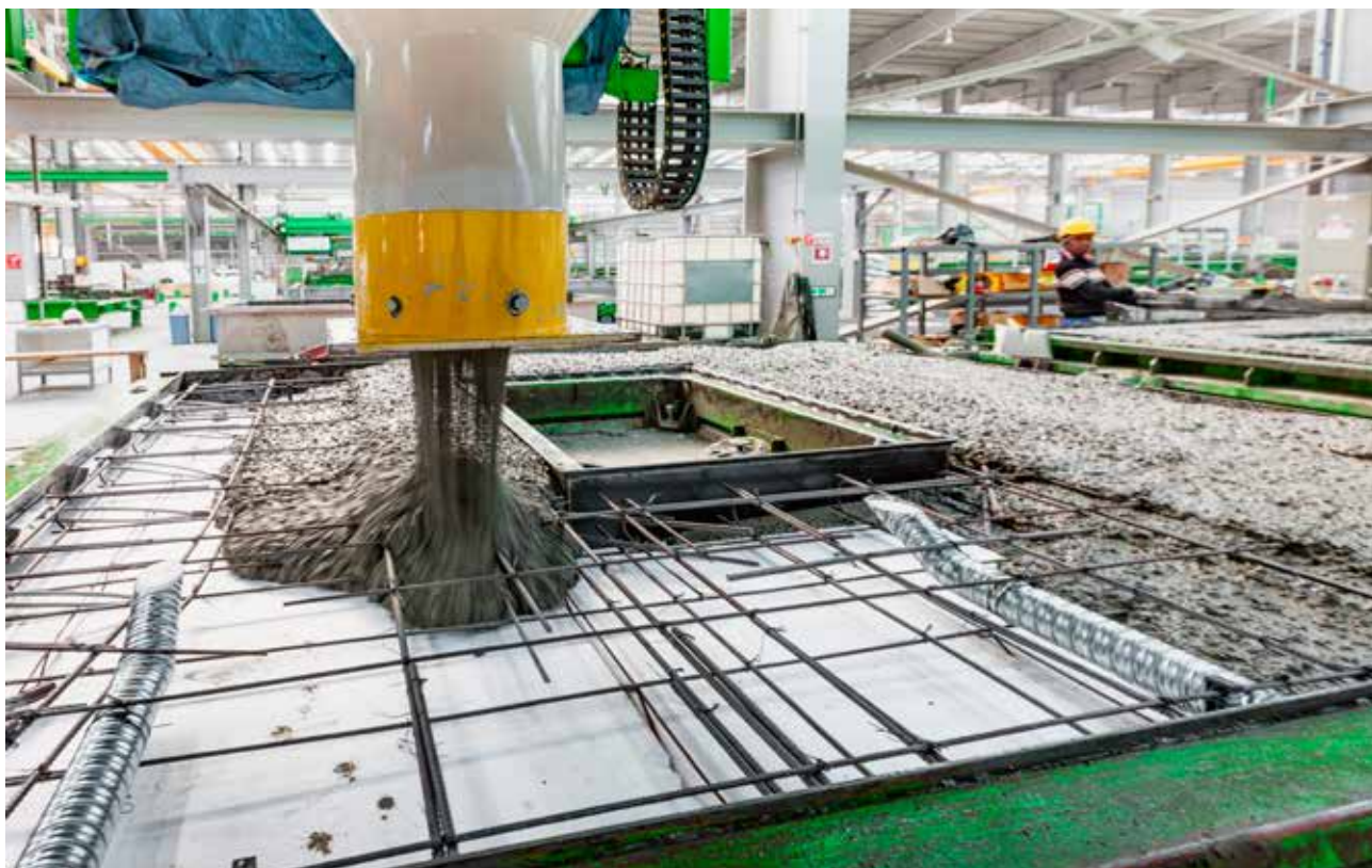
A wall panel being cast in an automated factory’s production line.
