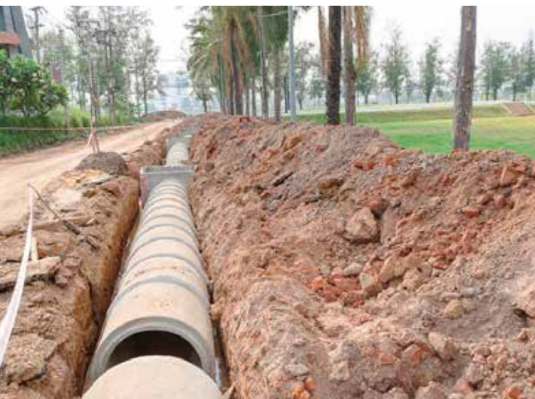
A culvert pipe installation.
