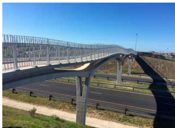
Innovation in concrete - Commendation – Pacaltsdorp Pedestrian Bridge.
