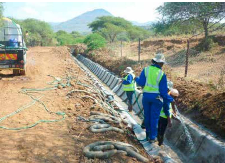
Hydration of the installed Concrete Canvas.
