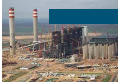
Kusile Power Station.
