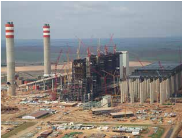
Infrastructure - Commendation – Kusile Power Station Main Civil and Completion Works.
