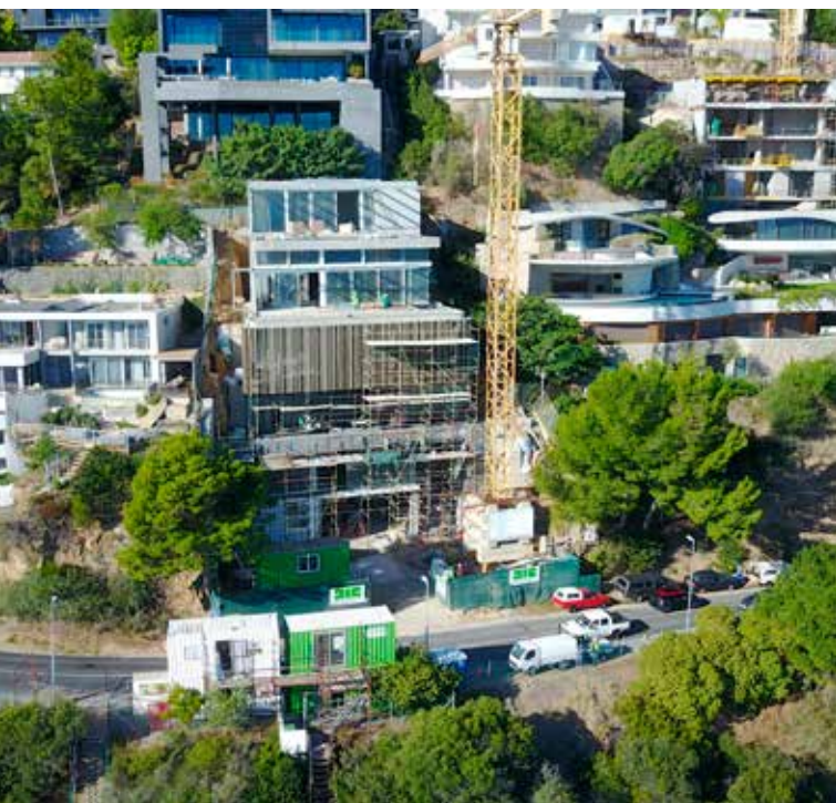
Development nearing completion with building structure supporting side walls.
