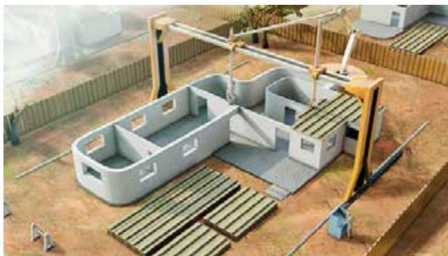
Contour Crafting Corporation's robotic 3D printer is designed for use where buildings need to be provided quickly and affordably (Copyright: Contour Crafting Corporation).
