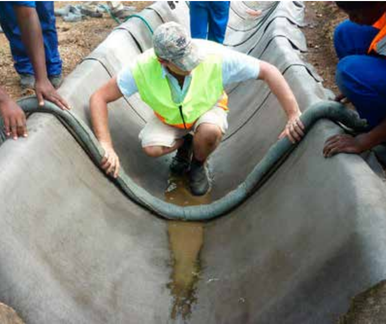
Concrete Canvas installed and overlaps weighted.
