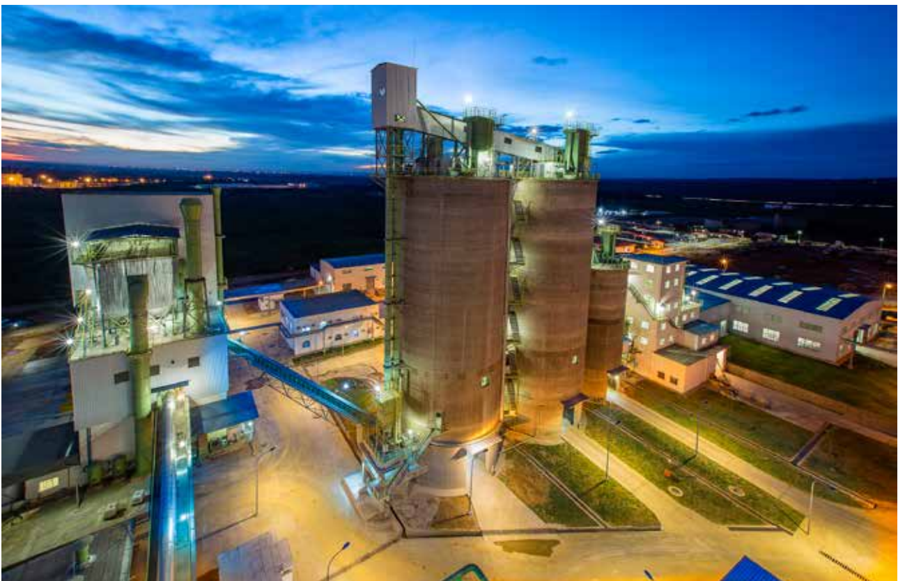
PPC's newly opened plant in Harare by night.
