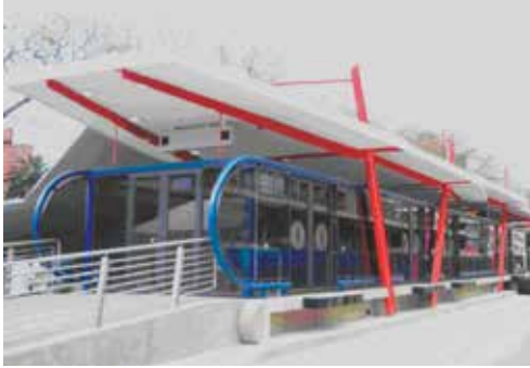
Johannesburg BRT building.
