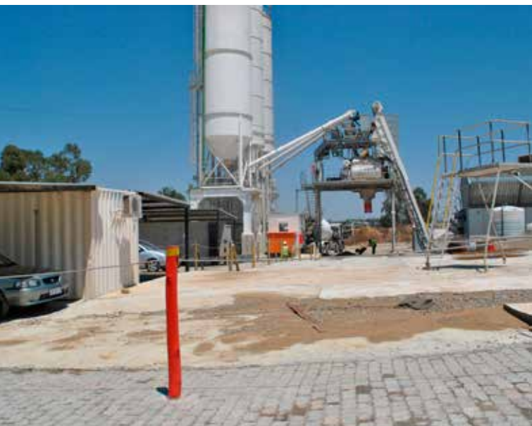
The return concrete has also been used around the readymix plant to pave large areas.
