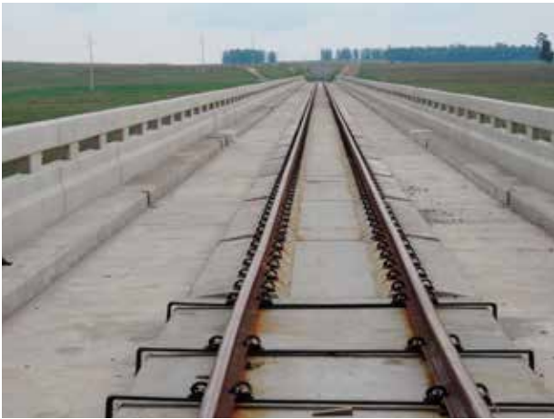
Innovation in concrete - Commendation – PY Track Slab.
