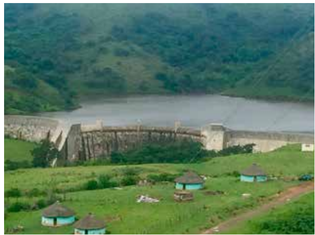
Infrastructure - Commendation – Mndwaka Dam – Rubble Masonry Multiple-Arch Buttress Dam.
