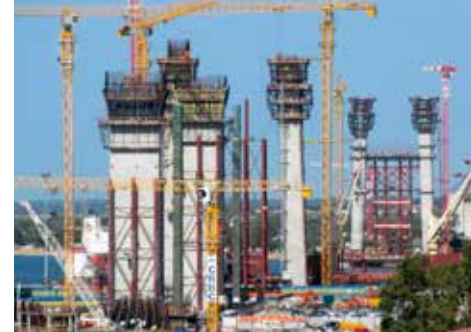
Maputo Bridge piers.
