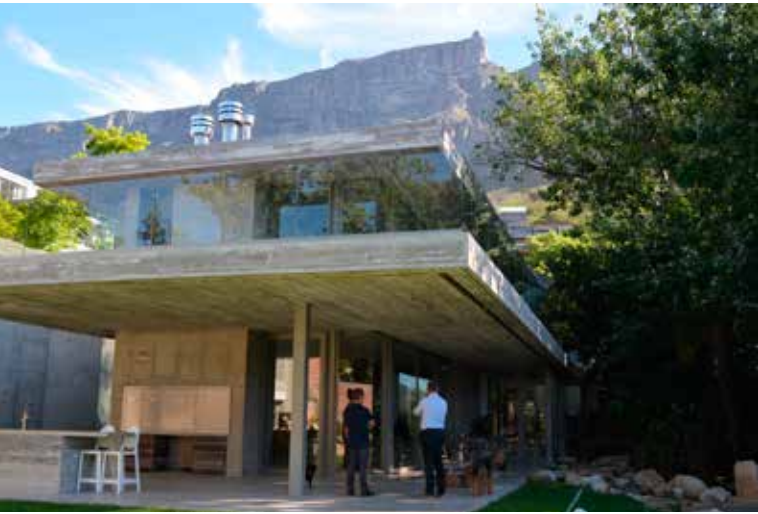
Buildings up to three storeys - Winner: Glen Crescent House.
