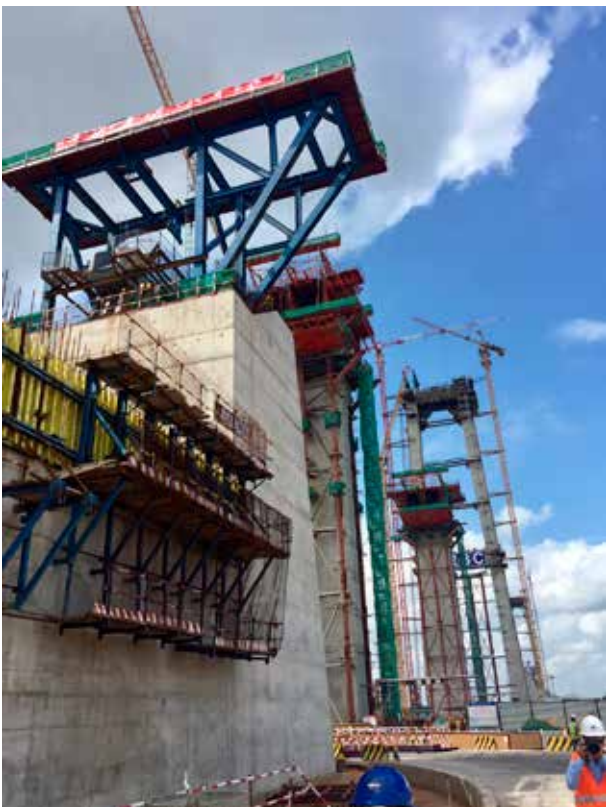
Infrastructure - Commendation – Concrete for Maputo Bridge.
