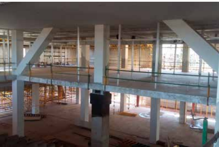
Buildings greater than three storeys - Winner: Sol Plaatje University Library.
