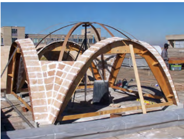
Cement-stabilised soil bricks were used to construct the dome.
