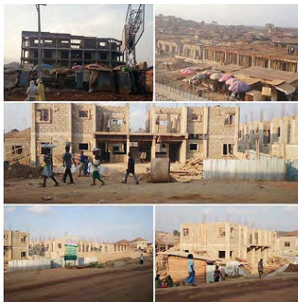
Construction of shopping facilities is ongoing all over Ogun State.
