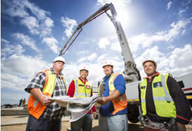
AfriSam's Centre of Product Excellence in Roodepoort works closely with customers to develop and test products to ensure that they suit particular and specific applications.
