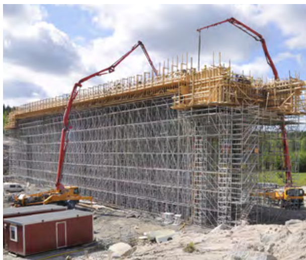
Concrete pumps place concrete into formwork supported by Layher's Allround system.
