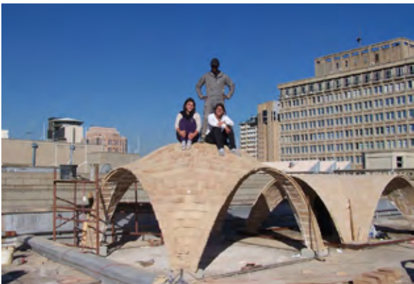
A prototype dome supports the weight of three adults.
