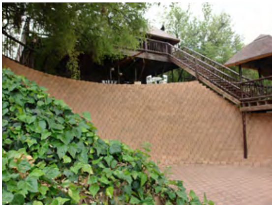
The Technicrete Earthform retaining wall built by Jannie Odendaal has weathered massive floods and emerged unscathed.
