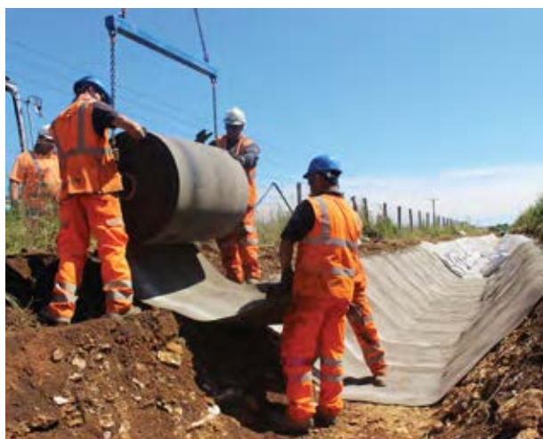
Concrete Canvas can be rapidly unrolled to form a channel lining.
