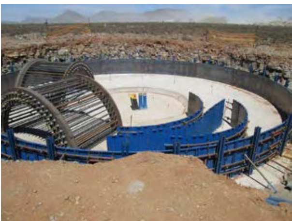
Foundation with electrical and communication cables in place.
