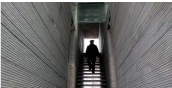
Inside the 3D printed apartment building.
