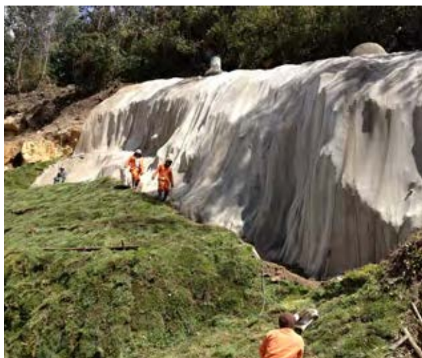
Concrete Canvas can be used to stabilise and protect slopes as a replacement for shotcrete and steel mesh.
