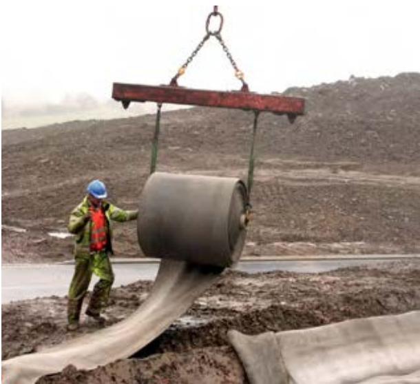
Concrete Canvas is significantly faster, easier and less expensive to install than conventional concrete channel lining.
