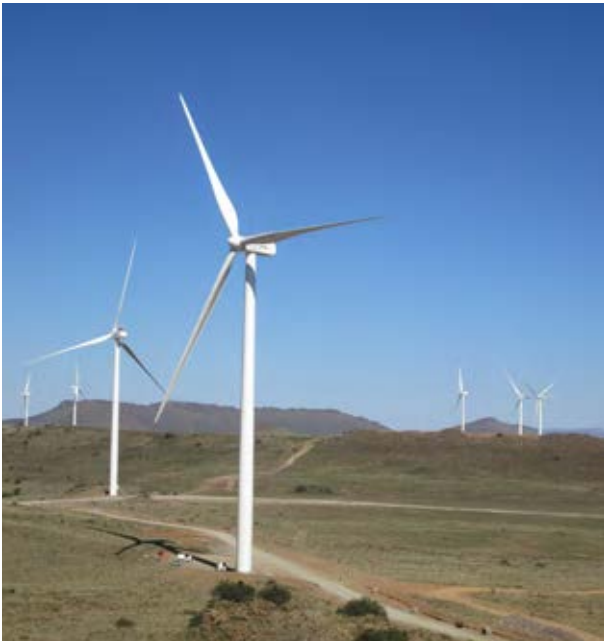
Noblesfontein Wind Farm's wind turbine generators stand 80 m tall.
