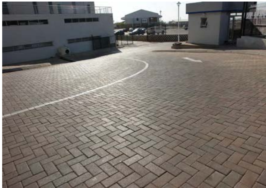
One of the seven Westvaal Delta car dealerships that had complete facility upgrades, including revamping petrol forecourts with Technicrete pavers.
