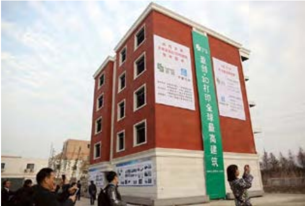
A five-storey building which has been 3D printed by WinSun.
