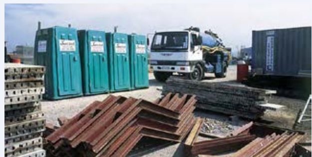
Sanitech provides its services to construction sites.
