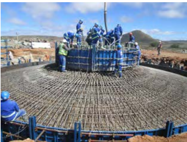
The foundation with its densely packed reinforcing.
