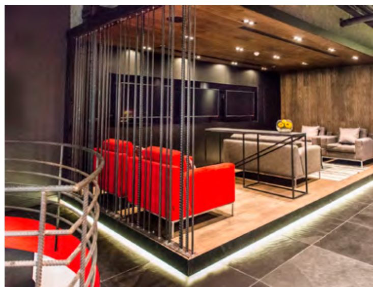
Common rebar has been used to create a screen and an innovative stair railing.
