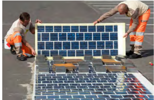
A trial stretch of road being laid with Colas' Wattway. The photovoltaic surface can bear the weight of six-axle trucks (Courtesy of Colas).
