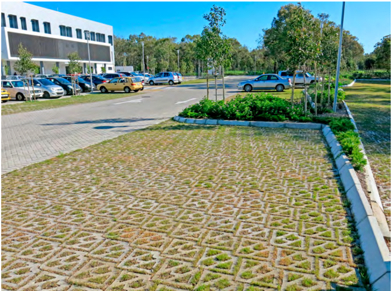
A Council directive required parking along Beach Road edges to be soft and green. Therefore Terracrete interlocking grass pavers were chosen.
