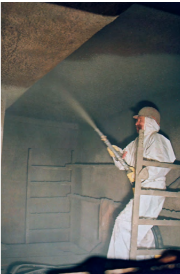
Sewament 10 being spray-applied.
