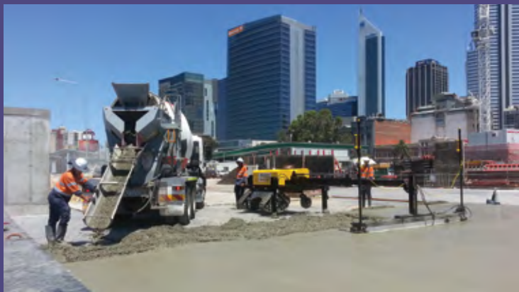
The Ligchine screed machine in action on a building site.
