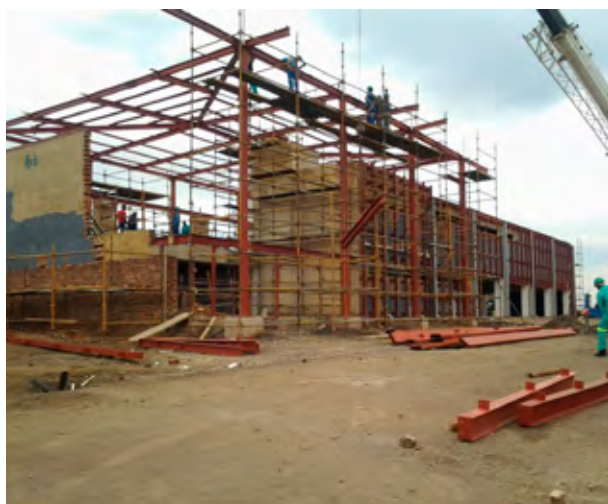
The Mercedes Advanced Driving Centre with alterations in progress.
