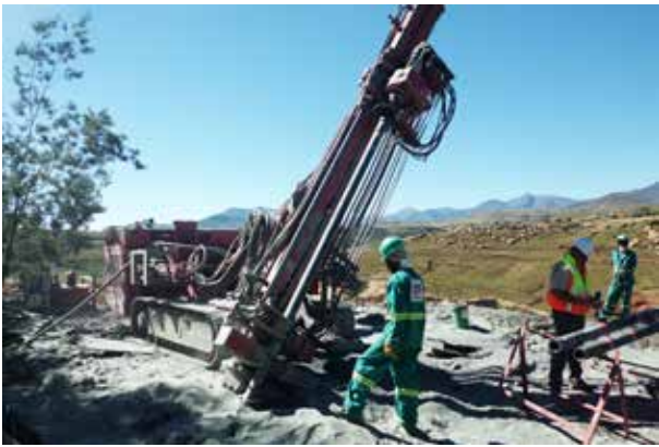
Drilling for rock anchors.
