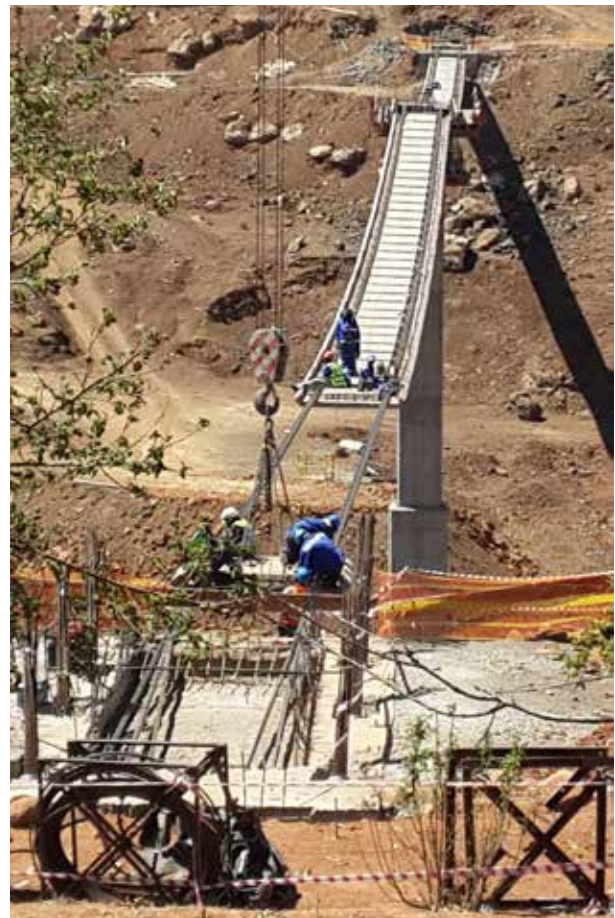
Launching of deck elements.
