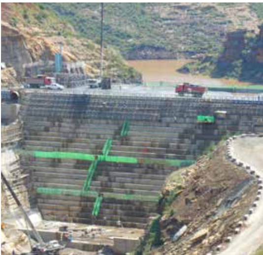
Metolong Dam outlet works.
