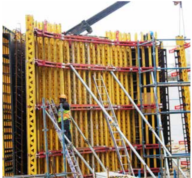
A ChrysoDem release agent being used on site.
