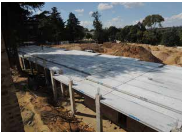
ESA hollow-core slabs forming the first floor of The Epic development.
