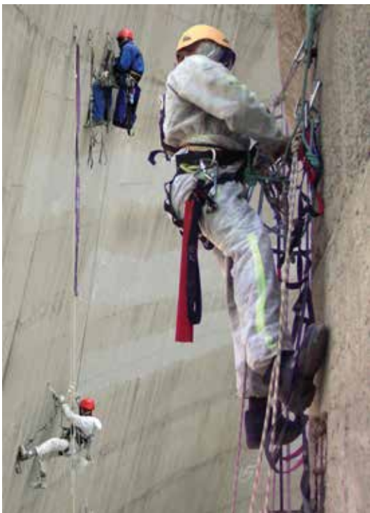
Skyriders team carrying out maintenance work on concrete.
