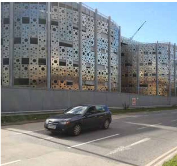
The multi-storey car park in Glasgow built extensively with precast concrete elements. (Photograph SCC Ltd).
