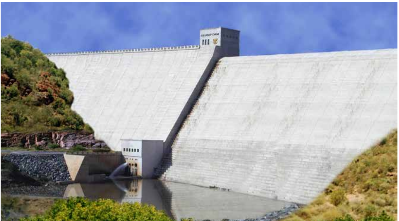
The De Hoop Dam's Vibratable RCC was a world-first use of Immersion Vibrated RCC.
