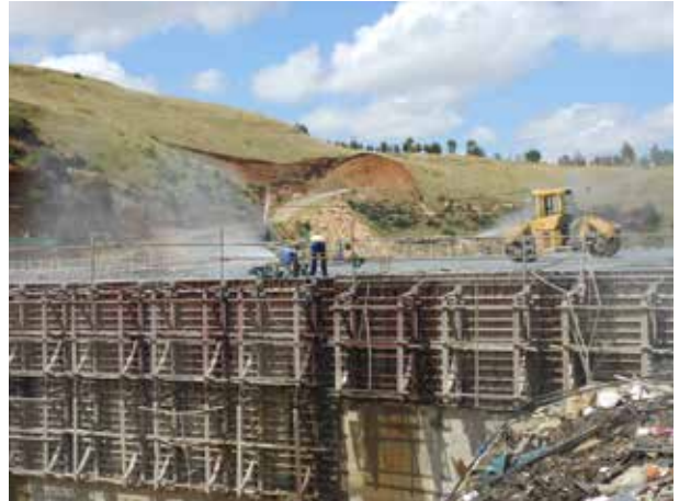
Shutters on the up-stream face of the Metolong Dam.
