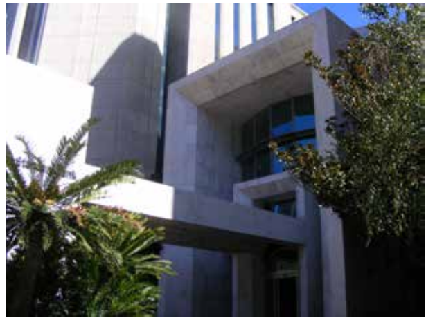
Marble arches at Standard Bank sprayed with polyurea on inside.
