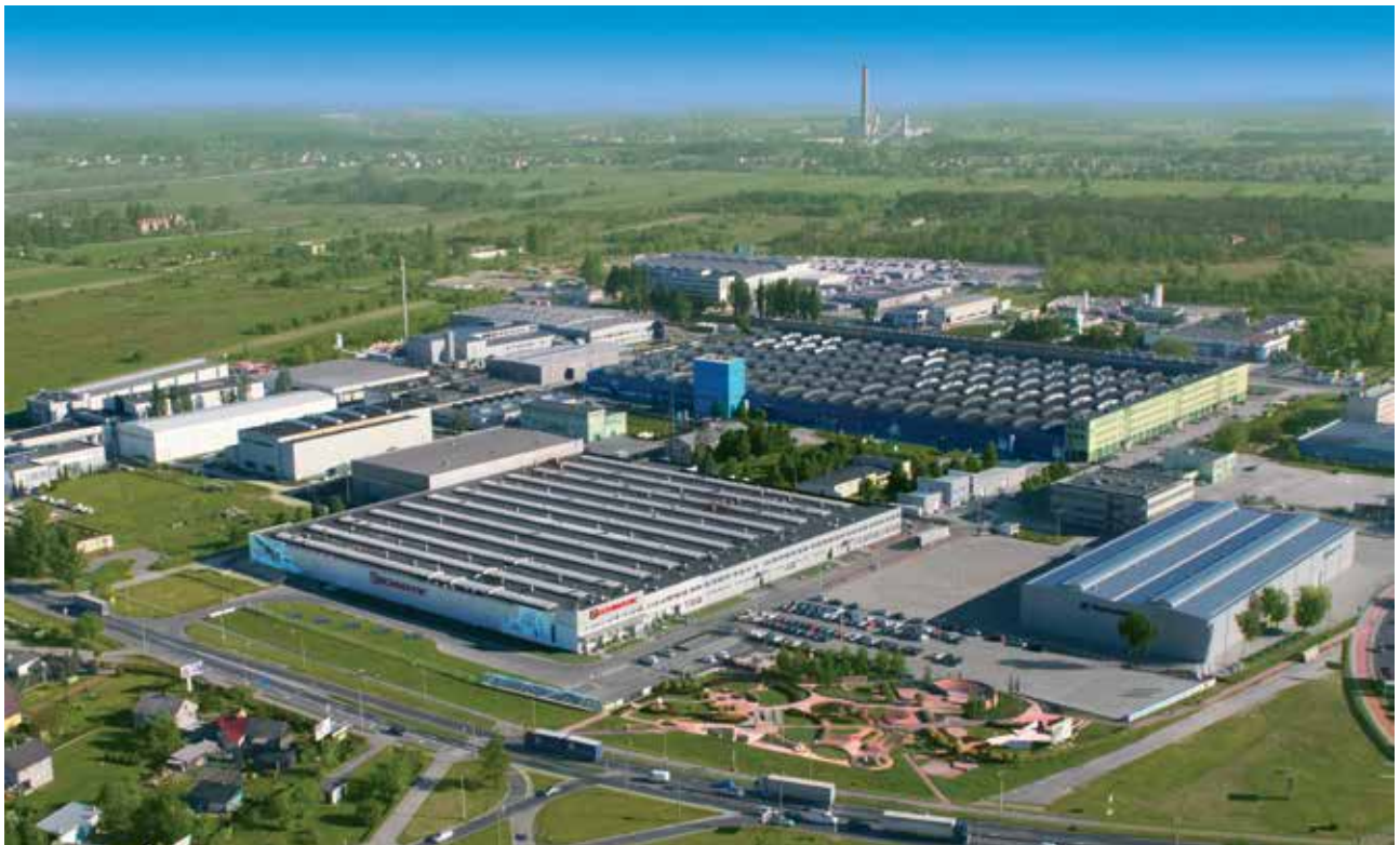
The new Techmatik plant in the Tarnobrzeg Special Economic Zone, Poland.
