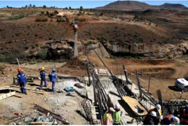
Launching precast deck elements using the main cables.
