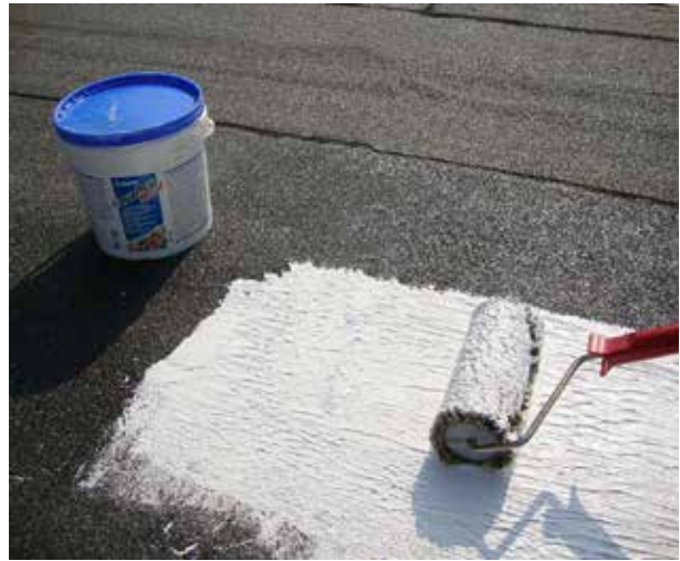
Aquaflex Roof HR is a ready-to-use waterproofing product with high solar reflectance.
