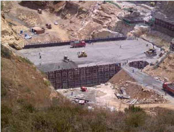
The massive wall of the Metolong Dam dwarfs construction vehicles.
