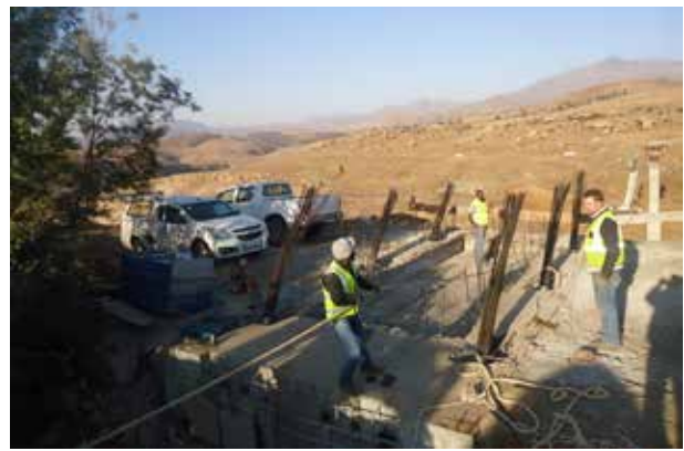
Stringing the main cables between abutments.
