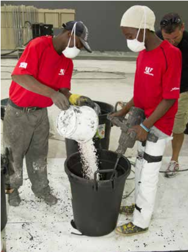
4.5-mm marble aggregate and 4.5-mm red aggregate being introduced into Stoneflow black matrix.
