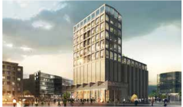
Pillowed glazing panels in the silo at the V&A Waterfront will bulge as if gently inflated.
