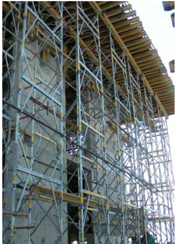
Staxo 40 and Dokaflex: a proven combination for high slabs.
