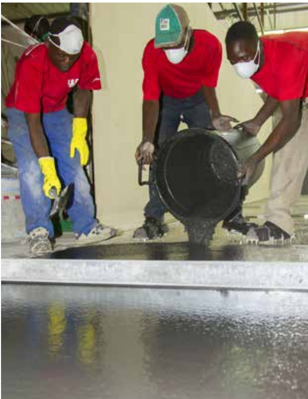
Mixed Stoneflow with marble aggregate being placed.
