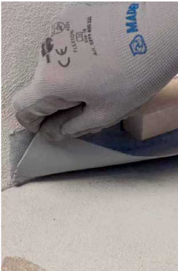
Mapeband SA has excellent adhesion to most substrates and gives immediate protection against heavy rain.
