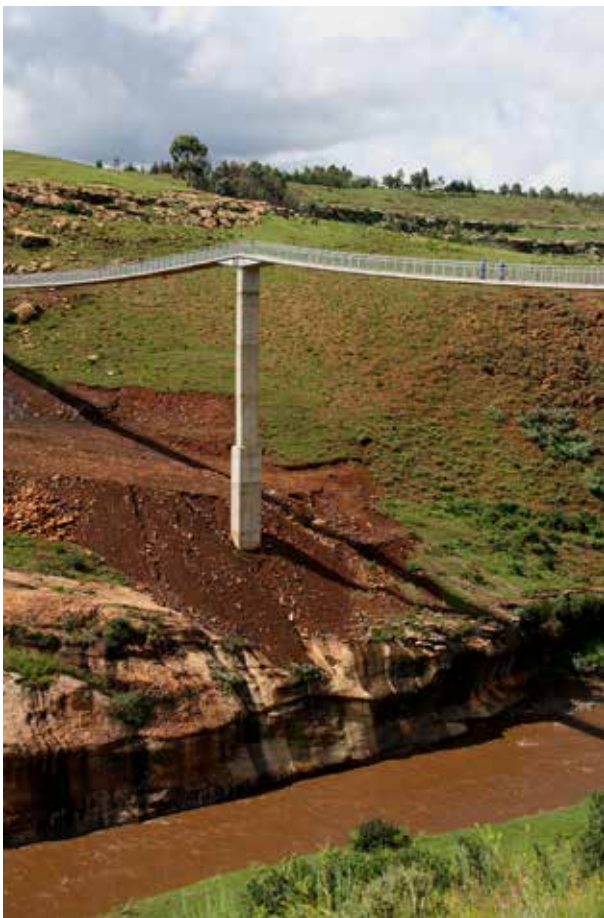
The completed Metolong Dam Pedestrian Bridge.
