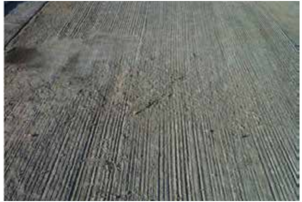
Alkali-activated concrete, City Deep container Terminal after 3 days.
