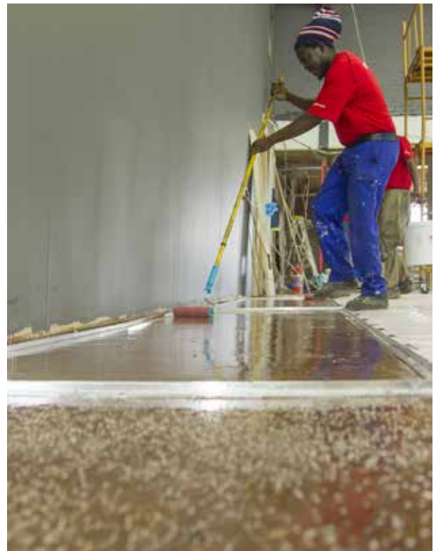
Priming coat being applied by roller with scatter sand aggregate
