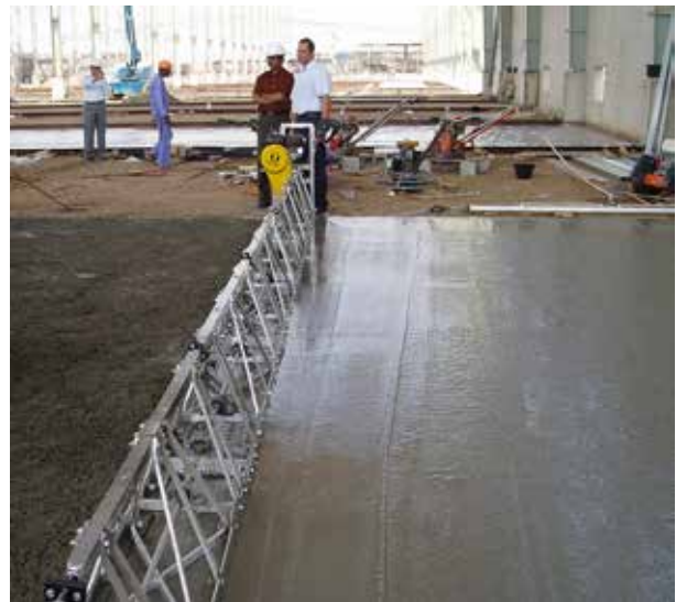
A concrete industrial floor under construction.
