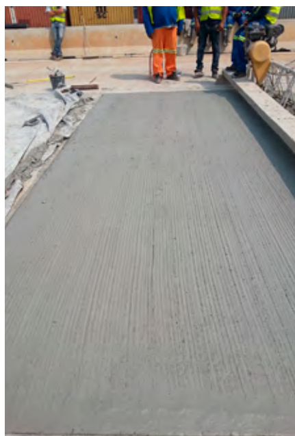
Casting geopolymer concrete at Transnet's City Deep Container Terminal in Johannesburg.
