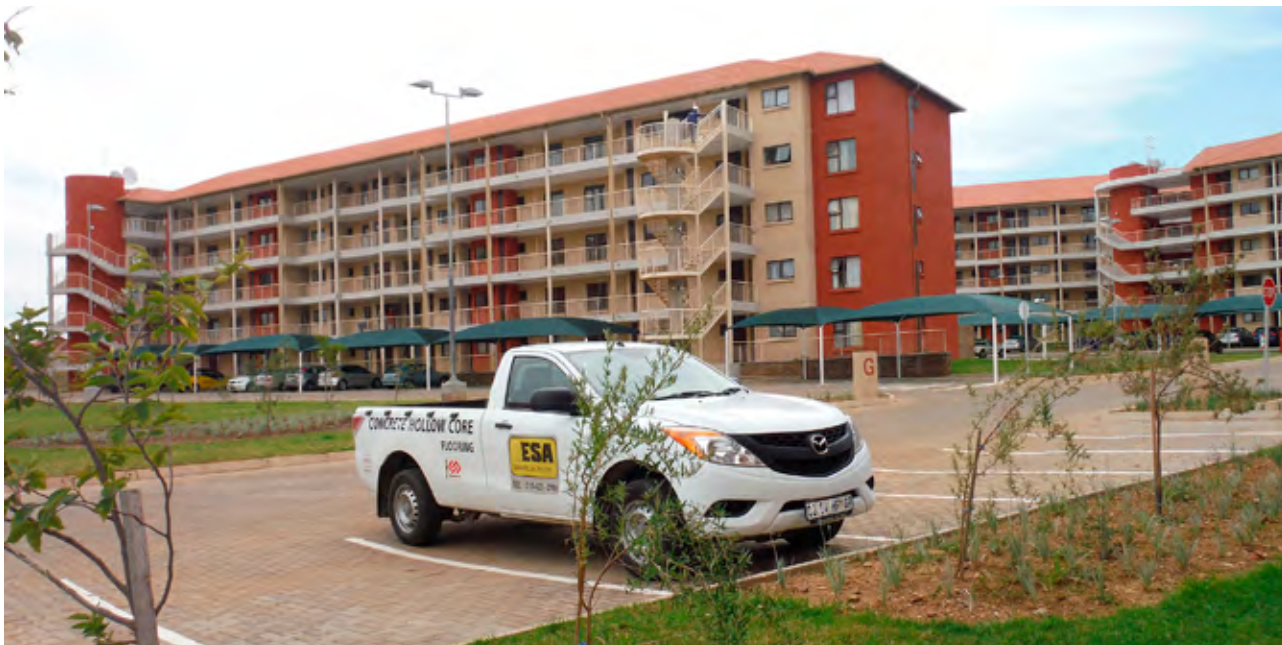
Using Elematic SA's hollow-core slabs reduced construction time by six months at Madeira Isles in Pretoria.
