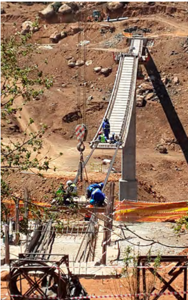
Launching the precast segments of the Metolong pedestrian bridge.
