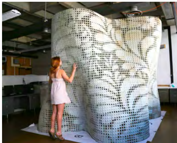
'Bloom' the 3D printed structure created by the University of California Berkeley.
