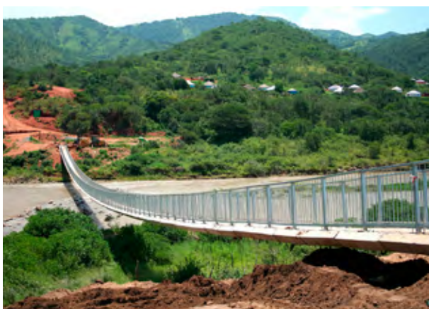
The completed Mkomaas River Bridge.
