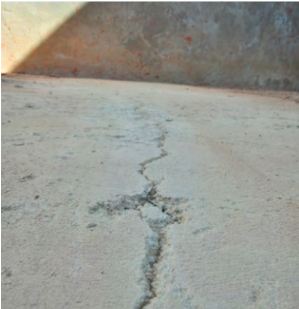
These pictures show examples of screeds on precast flooring slabs which have cracked due to an essential component, steel mesh, having been excluded during their construction.
