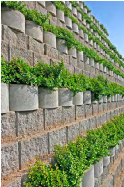
Waterwise plants soften a wall at the Al Jalila Children's Hospital, Dubai.
