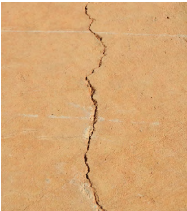
These pictures show examples of screeds on precast flooring slabs which have cracked due to an essential component, steel mesh, having been excluded during their construction.
