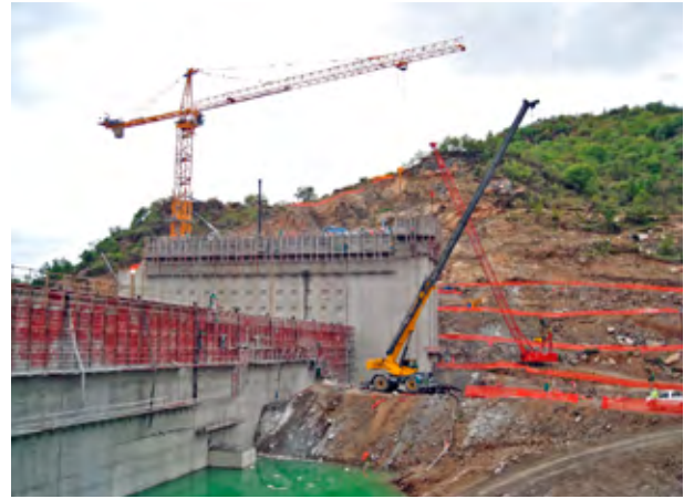
Potain tower cranes played an important materials handling role in the construction of De Hoop Dam.
