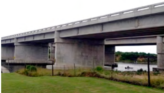
Rocla tailor-made the planks for the bridge to the customer's specification.
