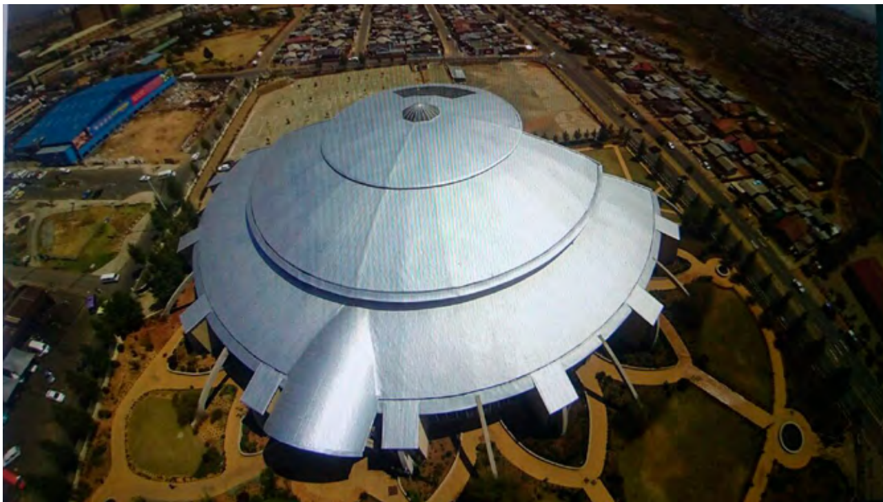
Multi-Dex 2000 recently refurbished the 9,000-m 2 roof of the UCKG church using Mapei products.
