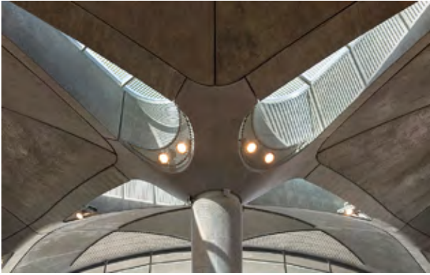
Concrete domes branch out from supporting columns like leaves of desert palms.
