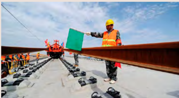
Railway construction operations
