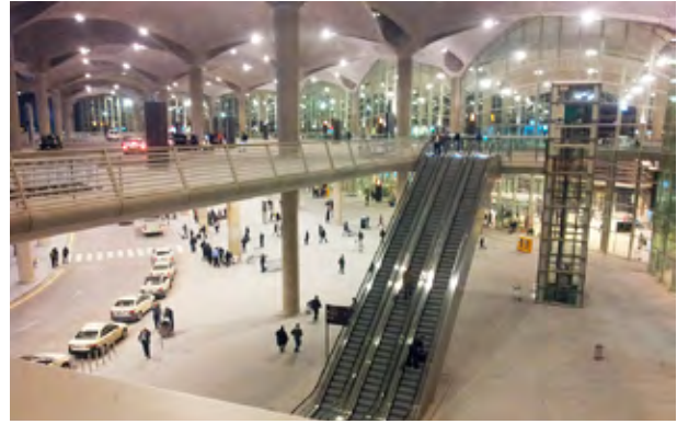
The dramatic concourse is glazed on all sides, allowing views of aircraft.
