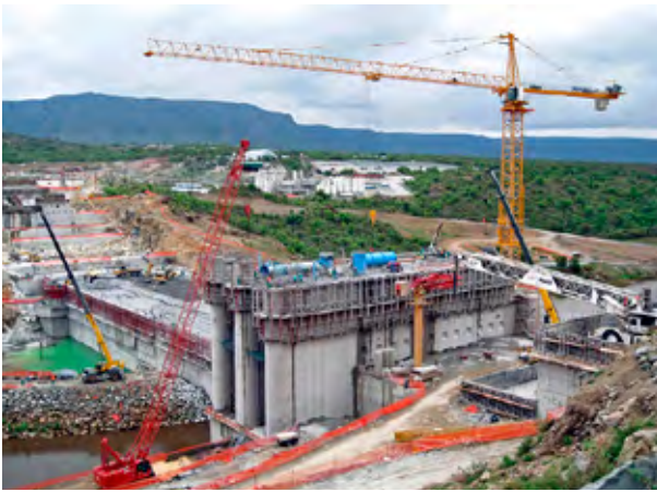
Potain tower cranes played an important materials handling role in the construction of De Hoop Dam.
