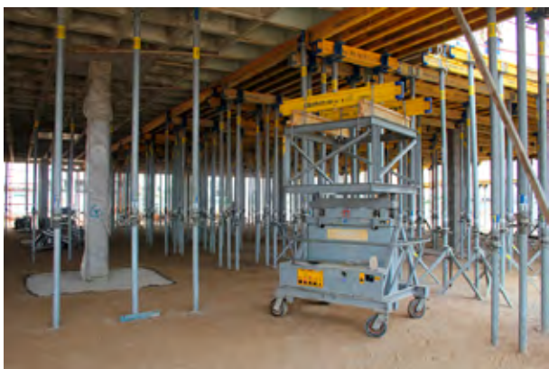
Shifting trolley makes light work of moving Tables as does the unrestricted access.
