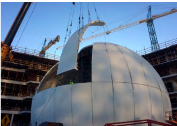
To maneuver the pieces, The Skanska team brought in a specialised 550-ton hydraulic crane with a superlift.
