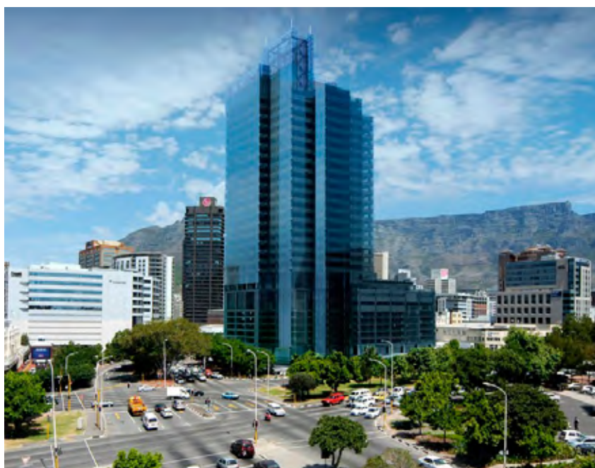
Mapei South Africa supplied admixtures to the Green star rated Portside building in Cape Town
