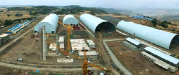
Construction of Dangote Ethiopia Cement plant at Muger in Ethiopia
