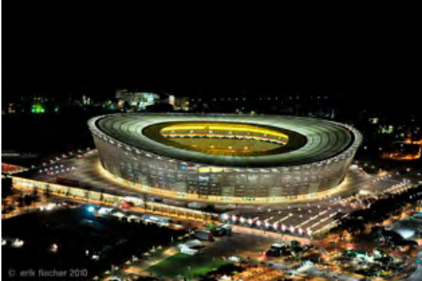
BASF provided 15,000 m 2 of Mastertop 1332 to Green Point stadium, Cape Town to enable floors to handle heavy foot traffic.
