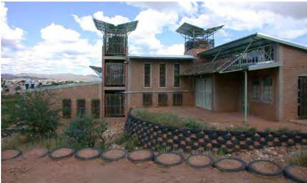
The Namibian Habitat Resource & Development Centre with its tyre retaining walls, rooftop solar installation and downdraft ventilation system.
