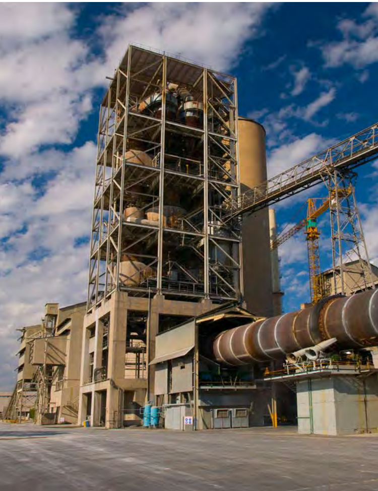
PPC's De Hoek plant is burning tyres to replace fossil fuel (coal) in their kiln.
