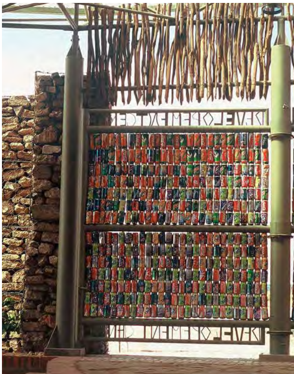
Old beverage cans were used to build attractive single-skin perimeter walls.
