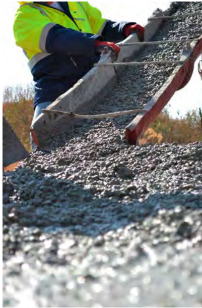
Construction in progress
