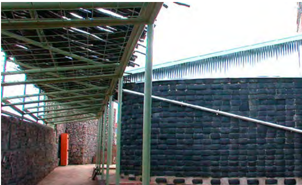
Walls and retaining walls were built with old car tyres.
