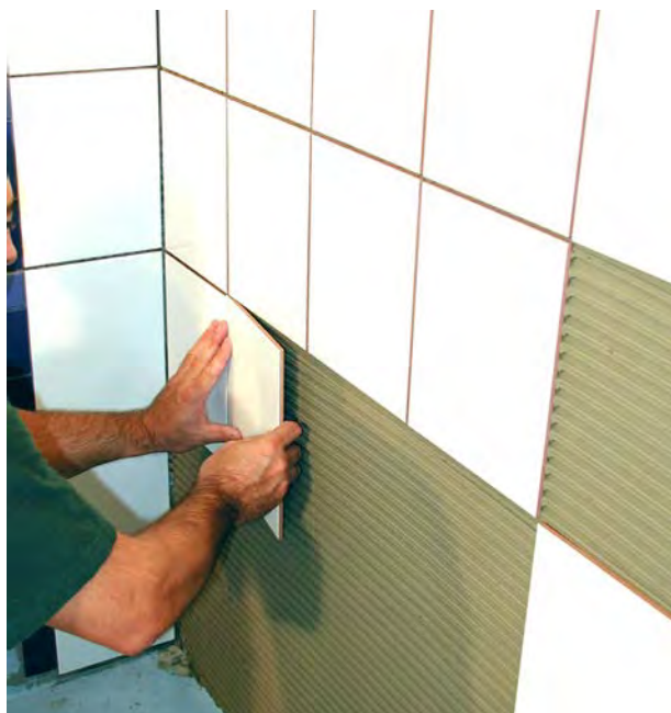
For high-quality, low-emission tile adhesives: with the aid of VINNAPAS®, even modern large-format or very thin tiles, and porcelain or natural stone materials, can be bonded reliably (photo: Wacker Chemie AG).
