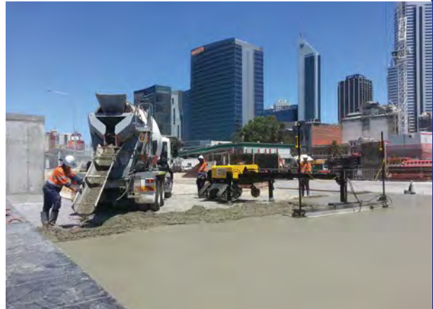
The Ligchine screed machine in action on a building site.
