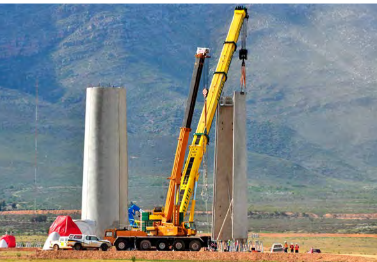
The Technical Excellence trophy went to Concrete Units for their innovative precast wind tower segments at the Gouda Wind Farm.
