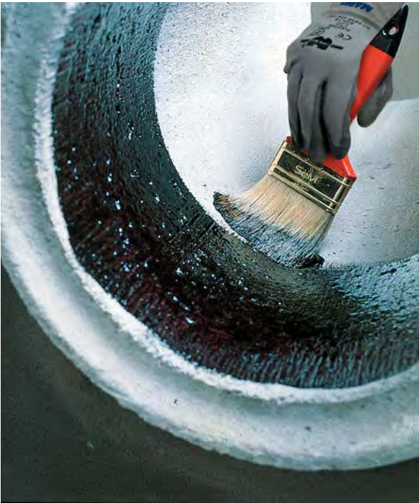
Duresil EB is an epoxy coating applied by hand to protect the substrate.
