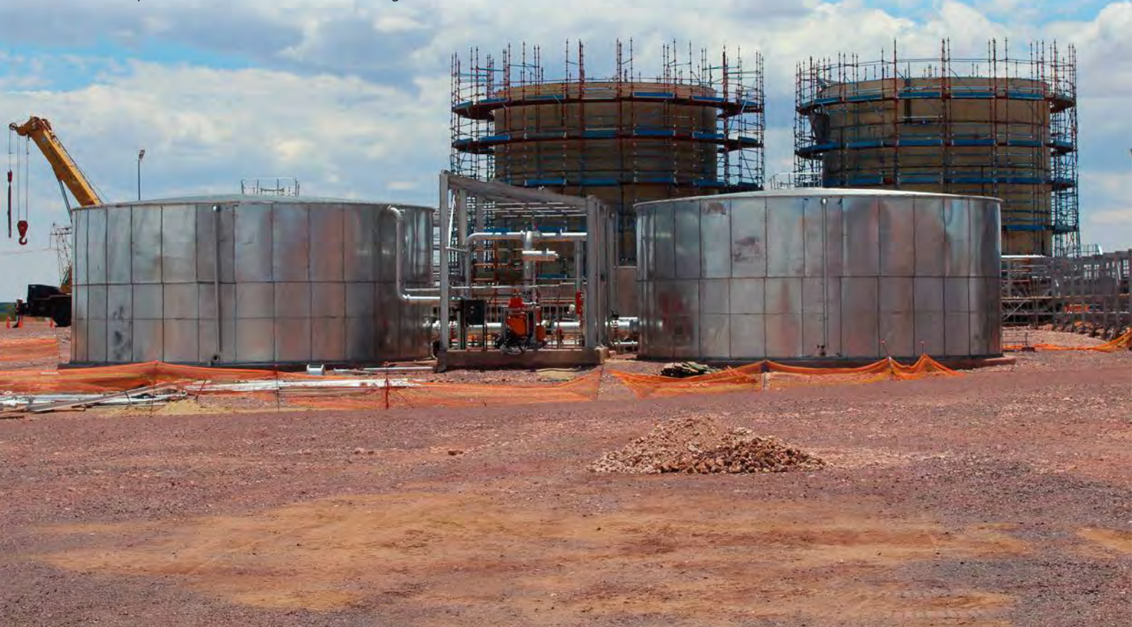
The ring beams were constructed to support the 1,500-KI diesel tanks.
