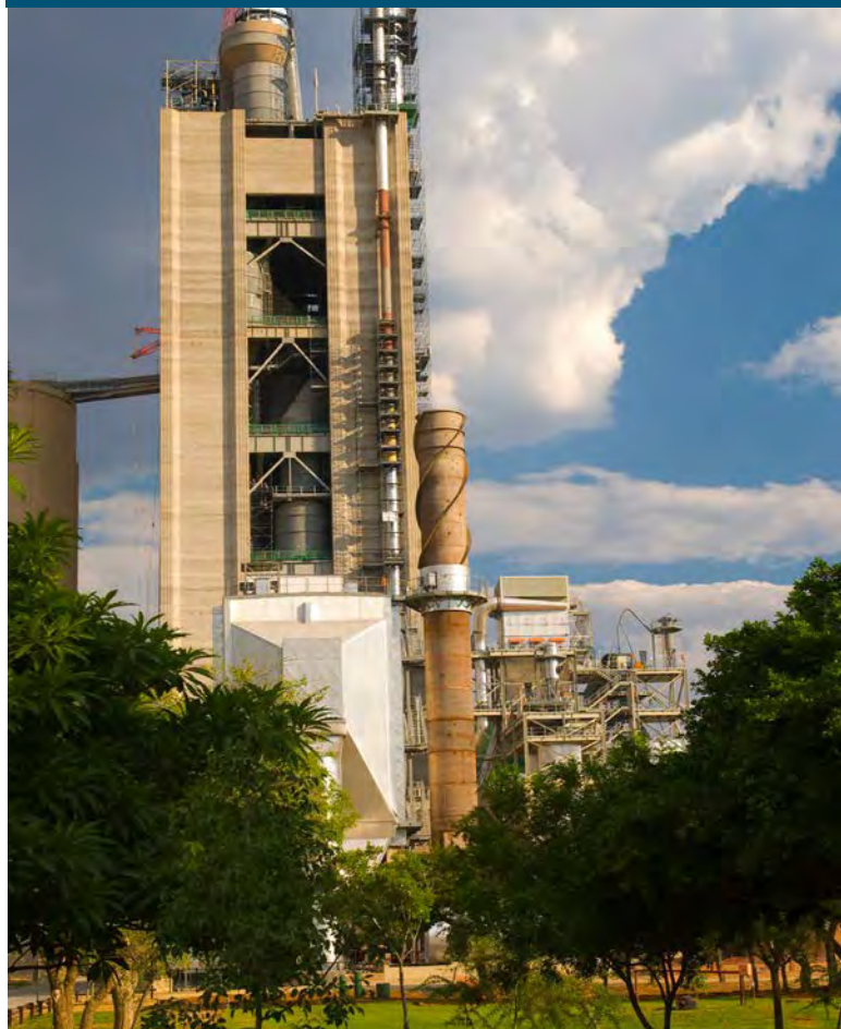
The Dwaalboom factory in Limpopo Province.
