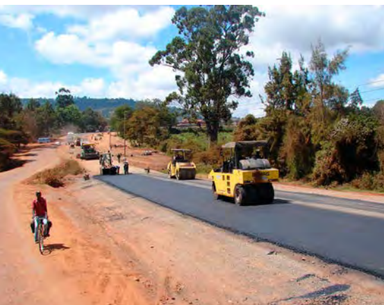
Road under construction in Kenya.
