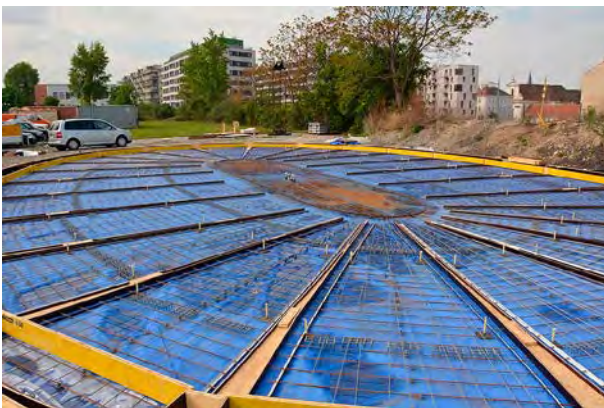
Flat rebar forms are laid out on top of a deflated plastic air cushion.
