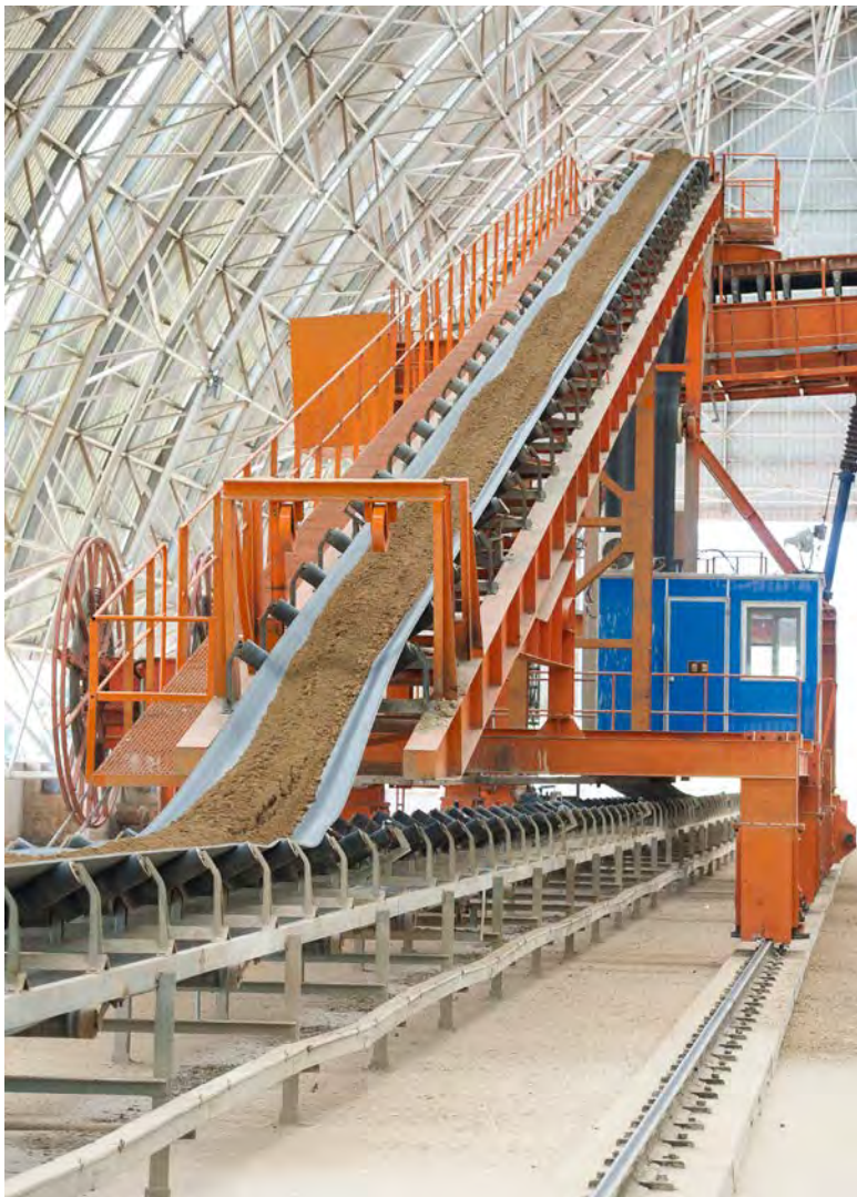
Inside the CIMERWA factory in Rwanda.
