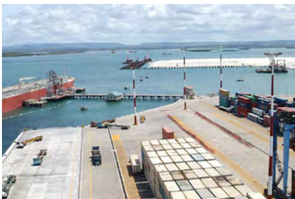
Berth 19 at Mombasa Port.
