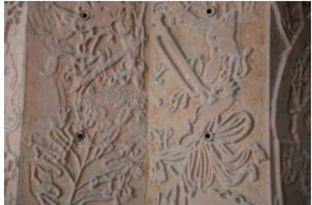
Drawings by Sara Fanelli formed the basis for form liners that capture very fine detail in pigmented concrete
