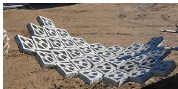
Mat lifted on two sides.
