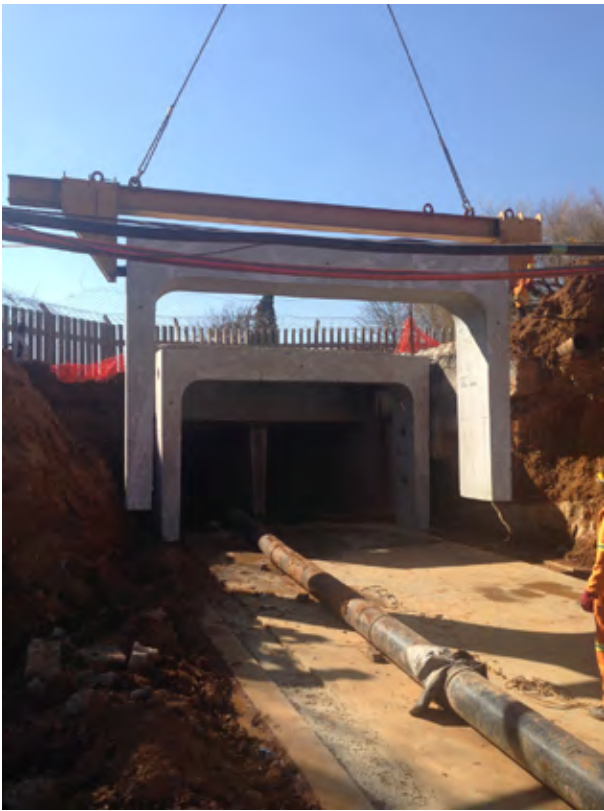
One of the mammoth culverts is lowered into position.
