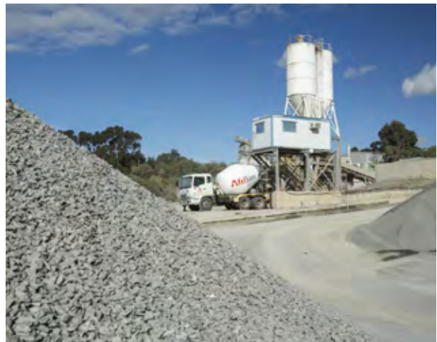
Each day AfriSam delivers an average of 3,000 tons of material to the project site.
