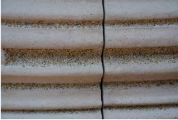
Bands of smooth concrete alternating with exposed aggregate concrete create some of the building's drama.
