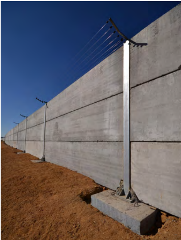
Electric security wiring was fastened to the steel supports.
