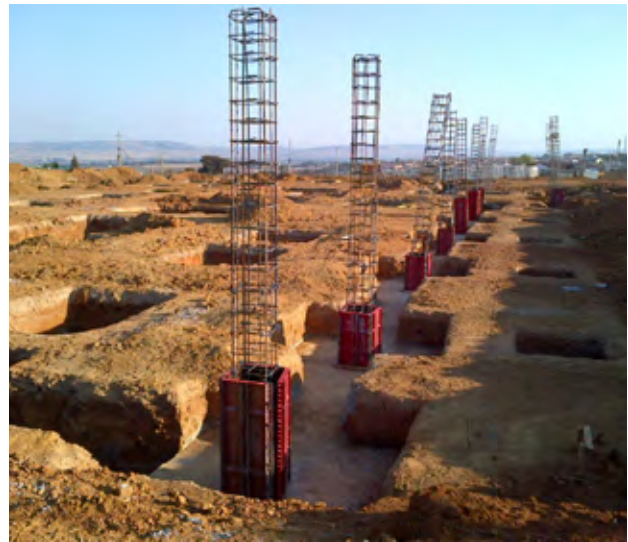
Constructing the foundations and raising support columns for the concrete roof.
