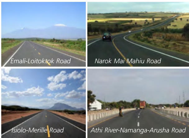
Four of the many current road construction projects in Kenya.
