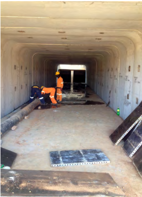
An internal view of the culvert channel.
