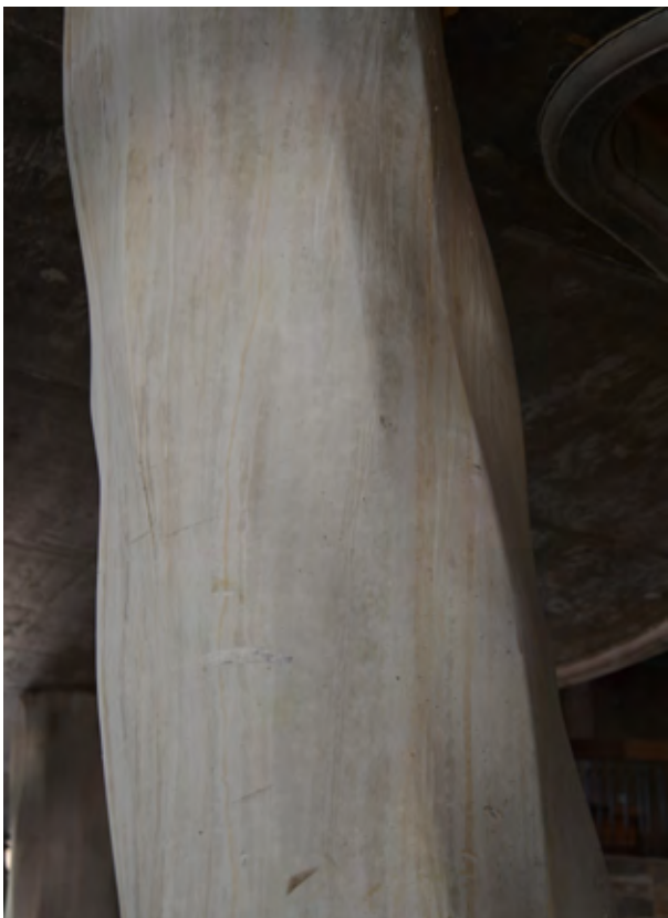
Form liners create undulating curves that “the pervert in each of us will want to touch”.
