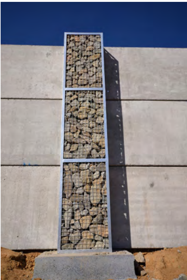
Cladding steel supporting columns with gabions added aesthetic appeal.
