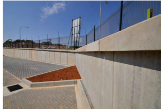
The completed Green Cross EGRW wall.
