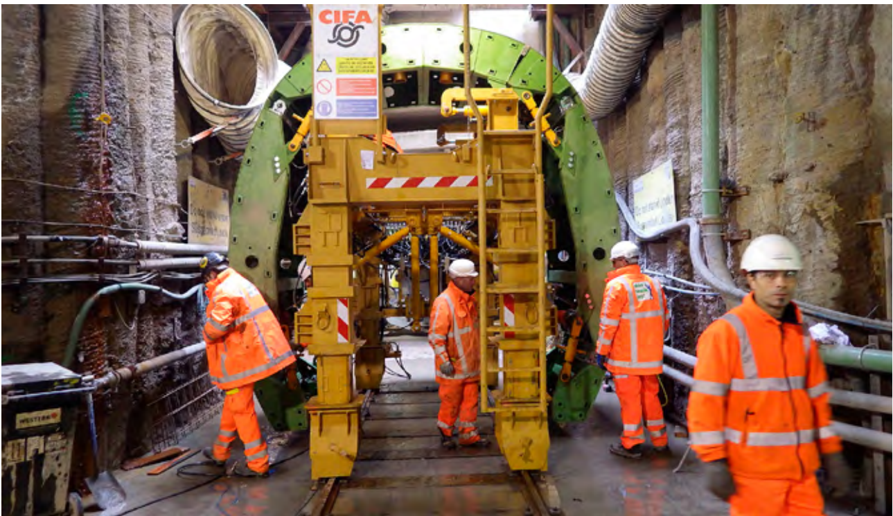
Travelling shutter installed in shaft.
