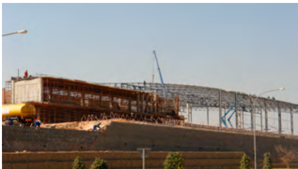
The Foschini warehousing building in the Lords View Industrial Park.
