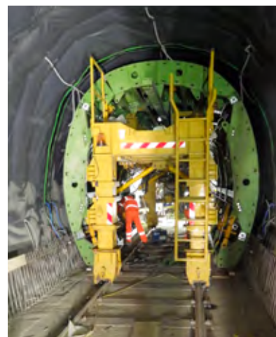
Page 26 - CIFA's innovative formwork solution for Victoria Station.
