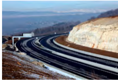
A section of Highway A41 North in France, built by Colas (Image courtesy of Colas)
