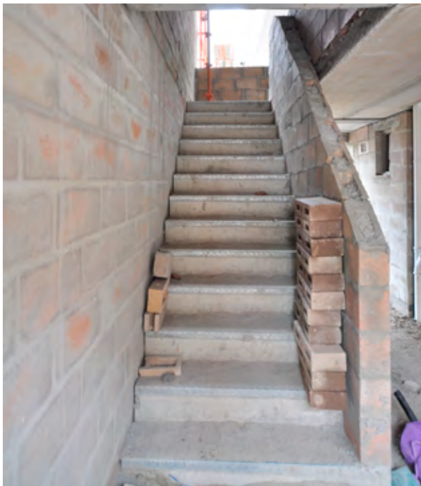
One of the precast staircases supplied by Topfloor.
