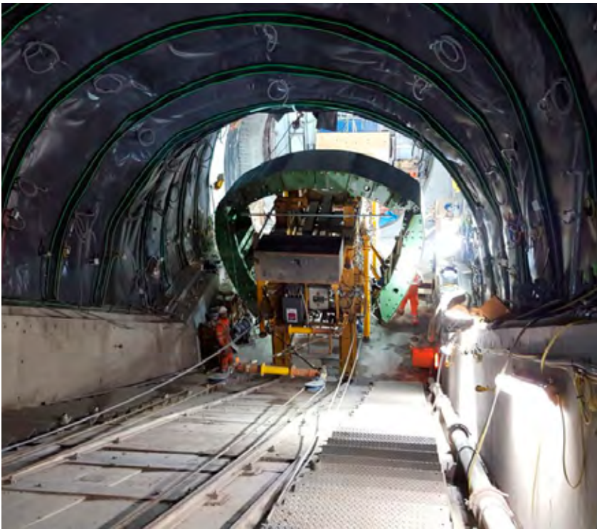
Pulling cables helped to position the travelling shutter.
