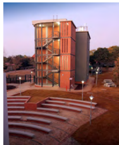
Page 28 - TuksSport High School built with a strong focus on preservation.
