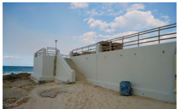
After Sika completed the repairs and coating.
