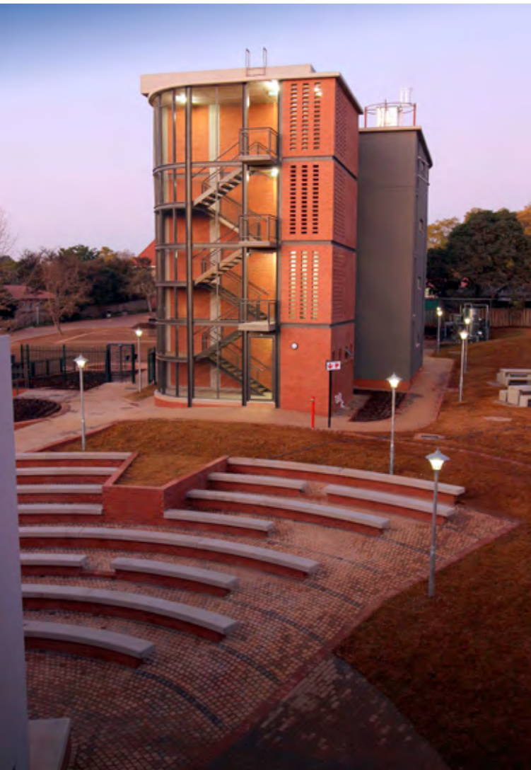
The four-storey residential block with the amphitheatre in the foreground. The curved steel fire escape was designed to soften the western red facebrick façade.
