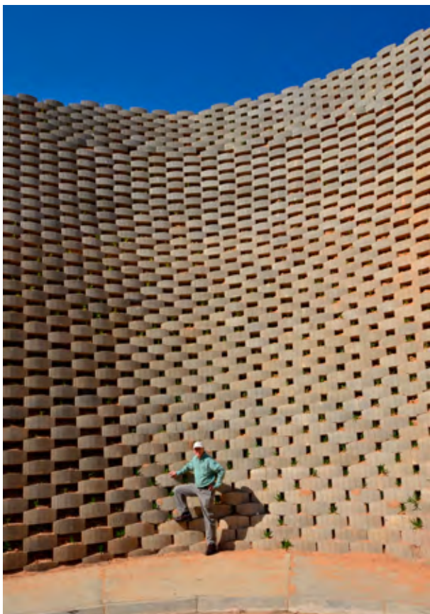
The 200m perimeter wall at its highest point of 12m.
