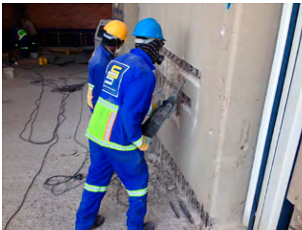
Sika breaking out concrete to rebar.
