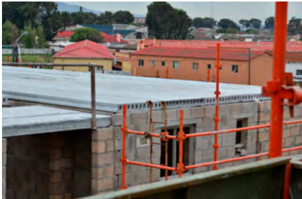
A close up of some Topfloor hollow-core slabs used at Lange.
