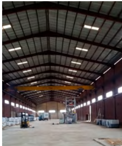
Sika's Nigeria plant under construction.
