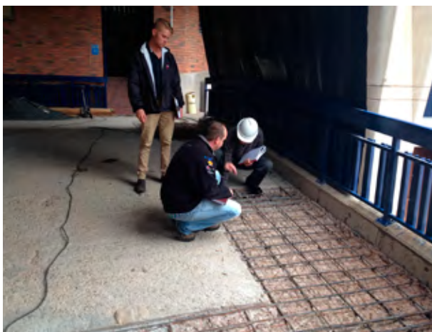
Final inspection, before repair material is placed.
