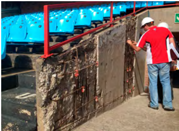
Sika inspecting exposed rebar.
