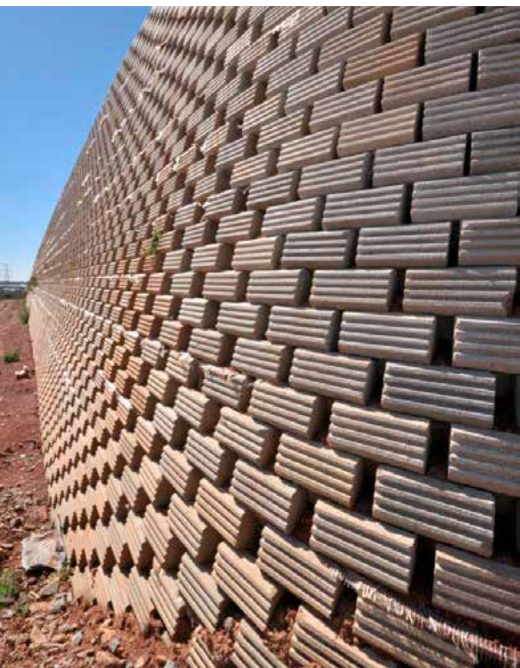
A portion of the completed wall in-fill.
