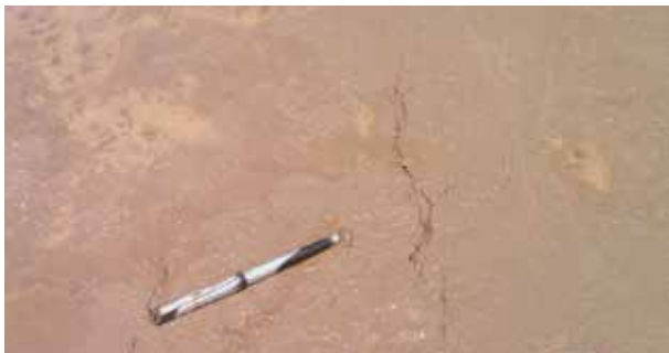
Plastic shrinkage cracking and plastic settlement cracking can, on occasion, penetrate the full depth of the slab. CHRYSO Micro Fibres provide effective crack control in concrete during the pre-hardening phase.
