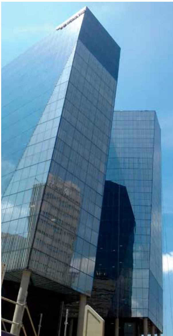
11 Alice Lane and its impressive glazed façade for which a.b.e. Construction Chemicals provided the structural glazing sealants.
