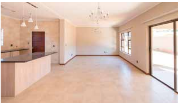
The living area in one of six new duplex cluster homes at Brandi-Ann residential estate in which the smooth-soffit finishes of Echo Floors' reinforced hollow-core slabs are attractively displayed.
