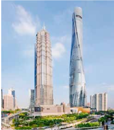
The Shanghai Tower has an elegant design that twists a full 120 degrees to mitigate the effects of punishing winds (Credit: Connie Zhou).
