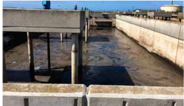
Aerators being emptied.
