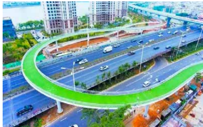
One of the cycleway's bridges (Xiamen Network)
