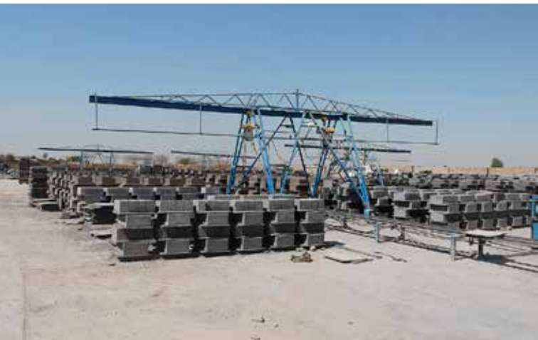
The UNI plant is capable of producing 17,000 standard bricks in a nine hour shift using skilled work.
