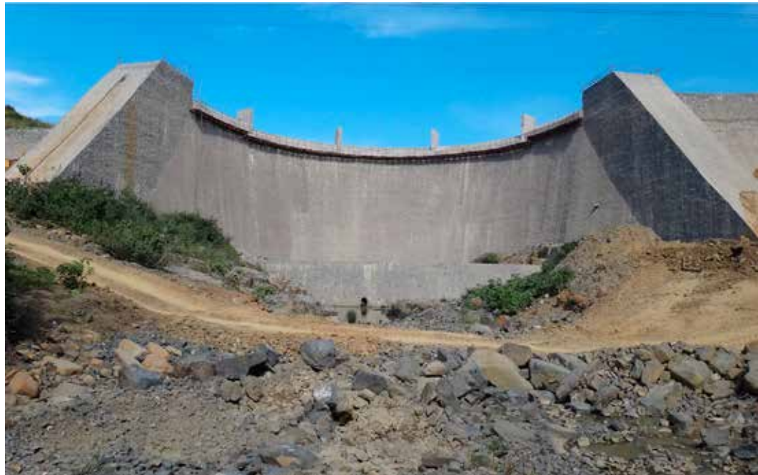
The curving lines of the Mndwaka Dam blend into the rolling hills of the Wild Coast. The Chryso SA Group provided several products for this Fulton Awards commended structure by Zana Manzi JV.
