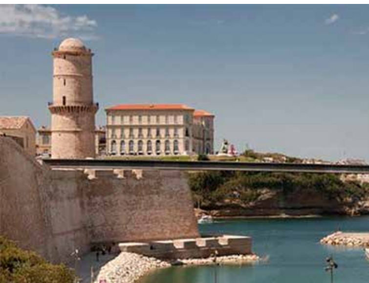
The 115-m ‘super-concrete’ pathway that leads to the MuCEM.
