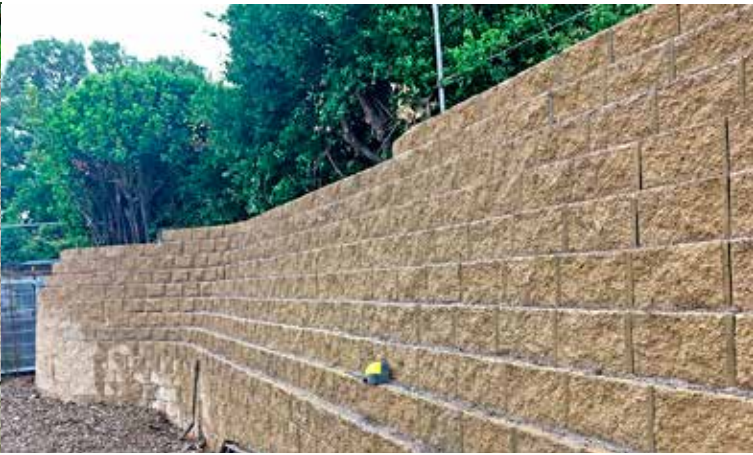
Ross Campbell Contractors erected this 4000-block wall in Rock, Cornwall.
