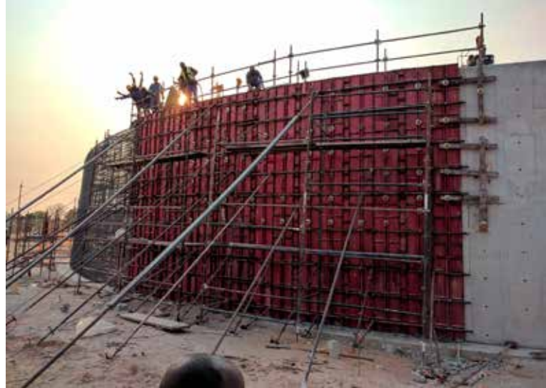
Finishing off a successful wall concrete cast.
