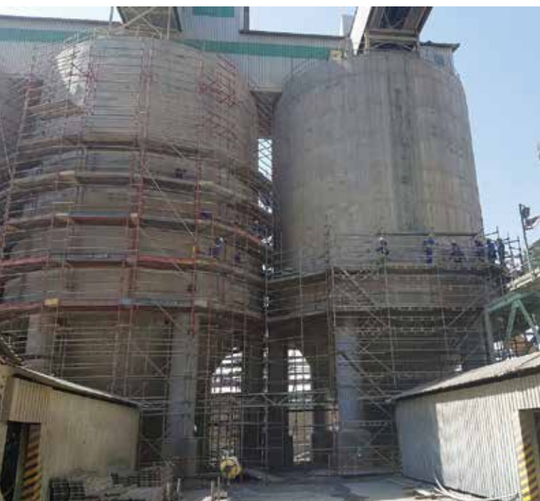
The installation of stressing tendons underway.
