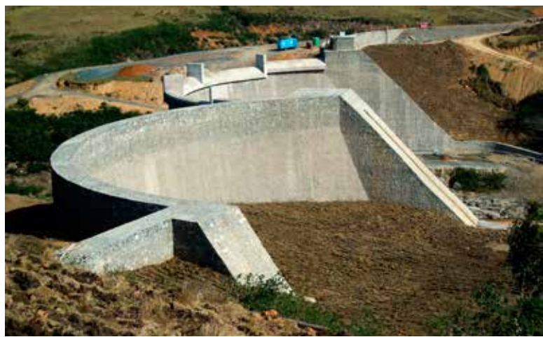
The construction of the RMC Mndwaka Dam provided abundant employment for residents of the isolated Wild Coast villages surrounding the dam. (Photo: CSSA).
