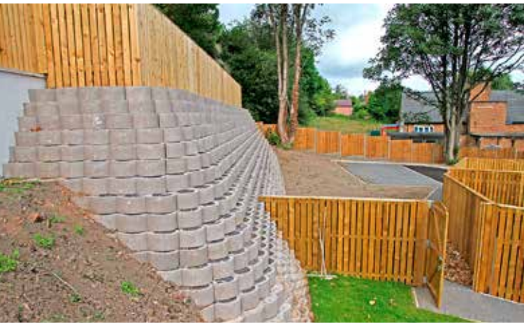
A Terraforce wall at Llwyn Onn residential complex in Holywell, Wales.
