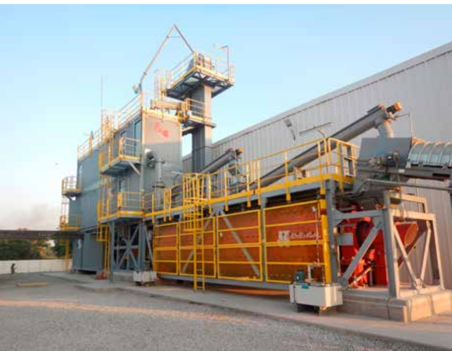
A Plug & Grind® installation for a client in Guatemala.
