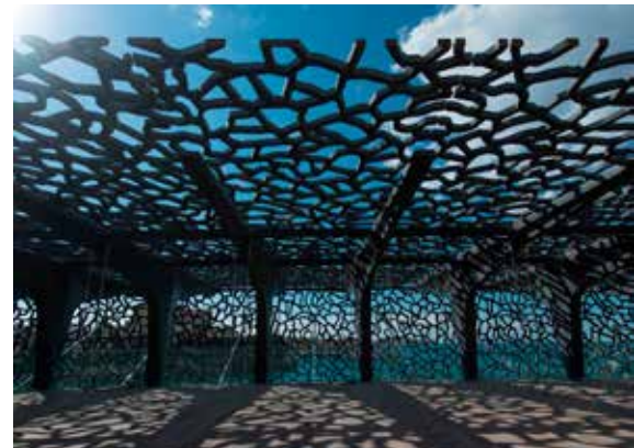
39 Ultra high performance fibre-reinforced concrete used at MuCEM.
