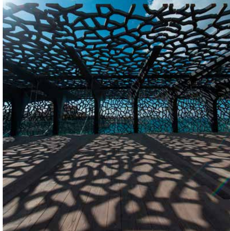
Ultra high performance fibre-reinforced concrete was used in the construction of the MuCEM.
