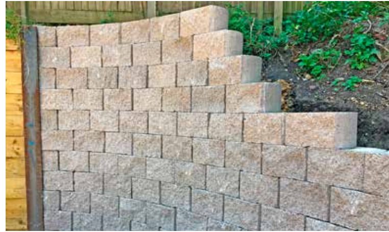
In Brill Terraforce blocks provided an affordable retaining wall for a cut slope.
