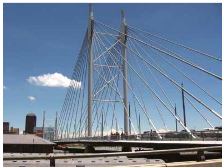
The iconic Nelson Mandela Bridge where Chryso admixtures were used.
