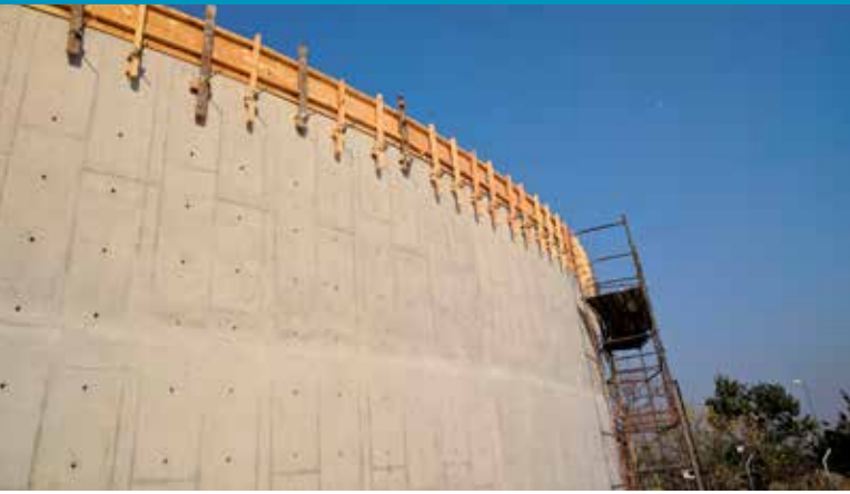
Erection of vertical formwork for roof ringbeam.
