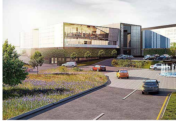
Anslow Park Phase 2, Bryanston.
